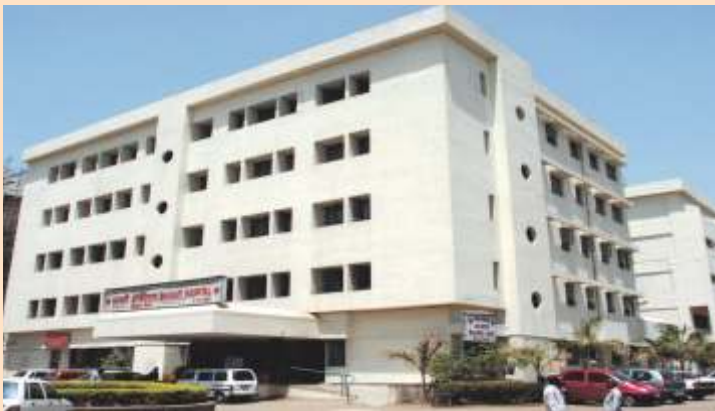
Bharati Hospital, Pune
