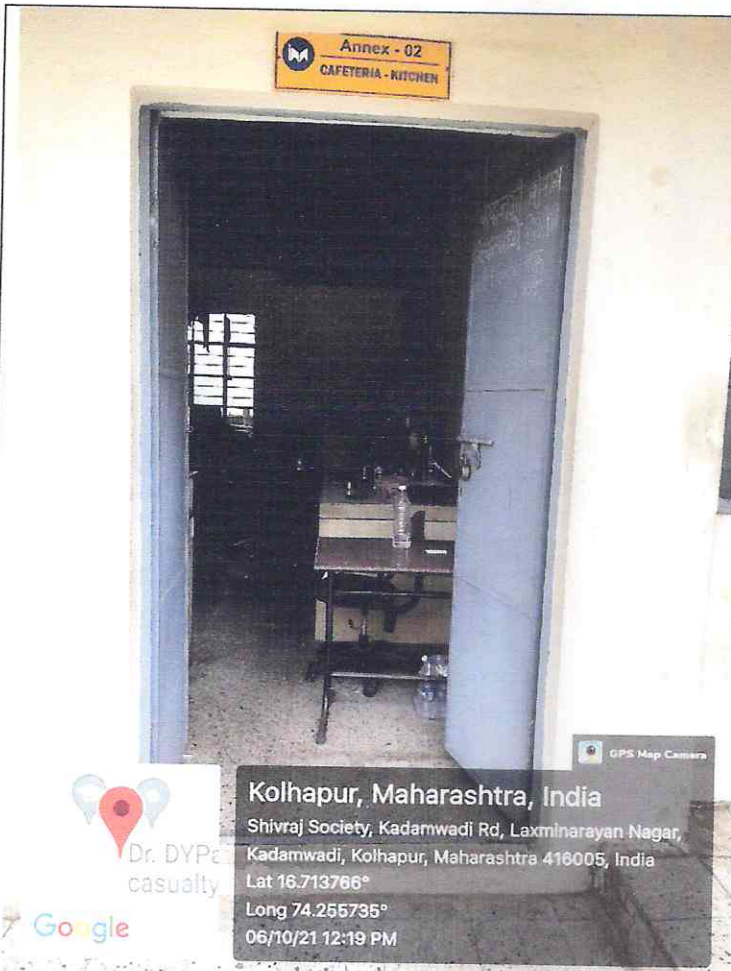
Annex-2 Cafeteria_kitchen Front View
