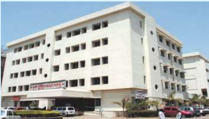
Bharati Hospital, Pune
