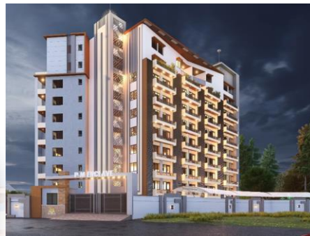
Group Housing at Darulsafa, Hazratganj
