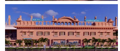
Gandhinagar Jaipur Railway Station, Jaipur IGBC Green Railway Station – ongoing project
