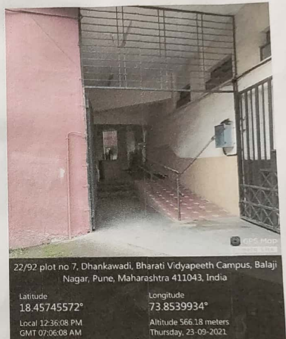
Figure 17: RAMP FACILITY IN THE COLLEGE
