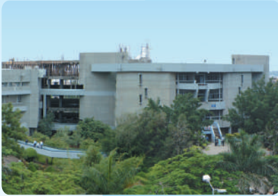
College of Engineering, Pune
